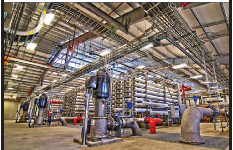
Hatch Mott MacDonald (No. 36) designed a 9.6-mgd reverse-osmosis water treatment plant, coupled with EPA Class 1 deep-injection wells to dispose of uranium-contaminated brine, for the city of Sterling, Colo. ■
