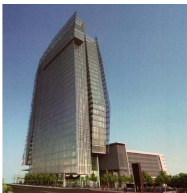
Crescent Communities - CRESCENT COMMUNITIE
